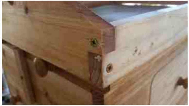
**Assemble Roof Beams and Gables using LONG screws in Pre-Drilled holes. Note Front and Rear Gables are slightly different**
