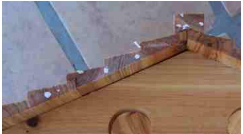
**Use 2 Long Screws to mount Roof Cap to Gable. Note the pattern of the Shingles to keep water out**
